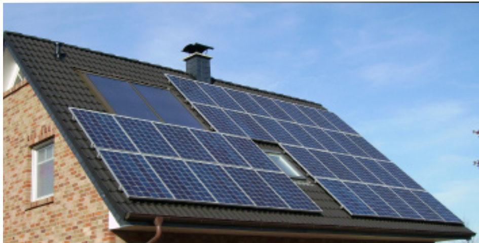
Distributed Generation: Solar panels on residential building roof
