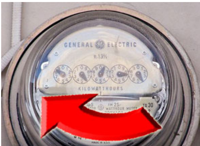
A net meter literally spins backwards when unused energy goes back on the grid
